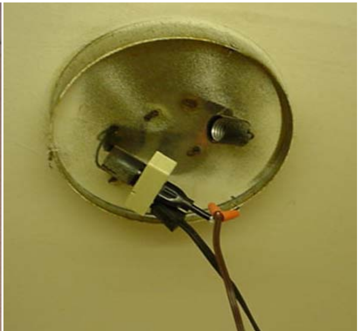
Flood light bulb too close to ceiling – fire hazard
