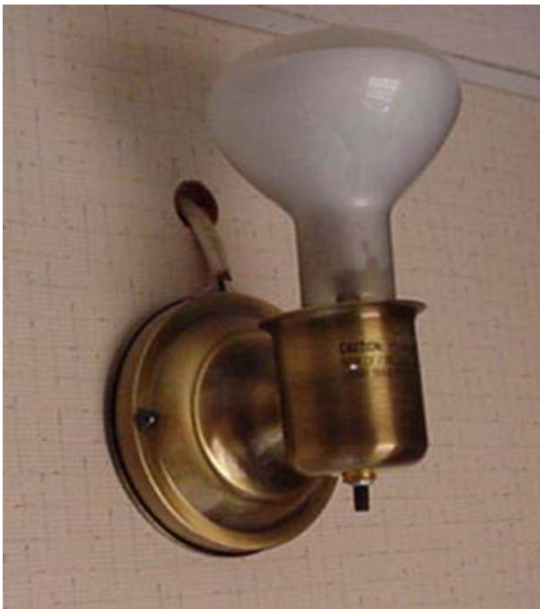
Flood light bulb too close to ceiling – fire hazard
